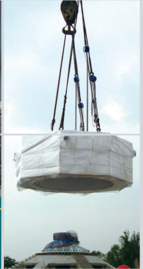
天线基座安装现场 ▲ Installation site of antenna base
